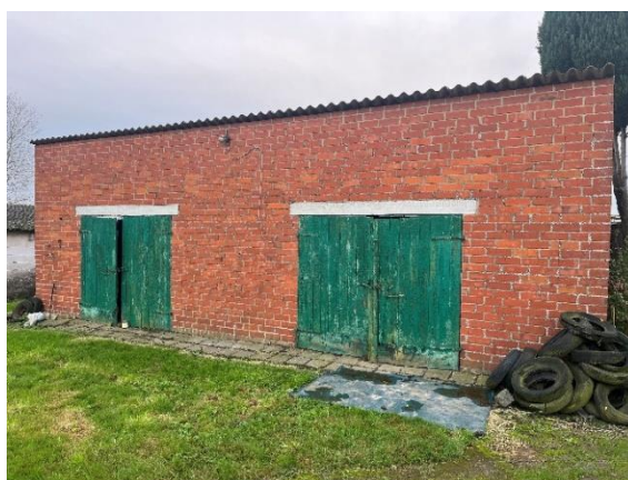
Stal 9 te slopen
