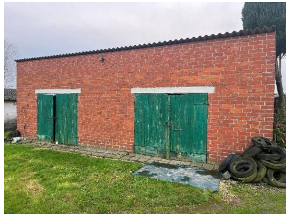
Stal 9 te slopen
